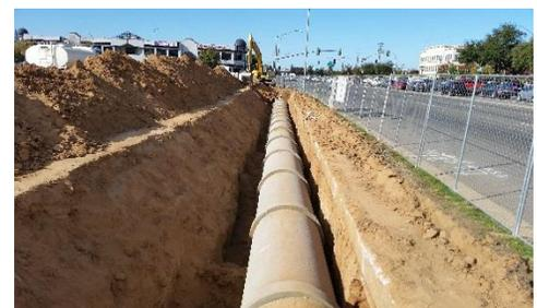
installed approximately 1,040 feet of RGRCP valued at approximately \$500k to relocate existing facilities (Victoria Colony (340'), Victoria (290') and Tracy (410')) for the California High Speed Rail project.
