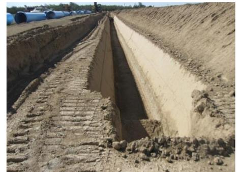
tendency to breach, and the cost of open canal maintenance. Also, by piping this section of canal, FID is able to provide better service to the water users as it eliminates service disruptions caused by canal breaches.
